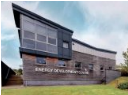
Energy Development Centre Quality industrial and workshop units
